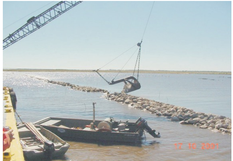
Rock being placed at Bayou Chevee.
