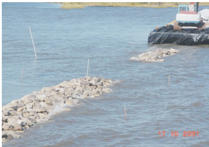
Rock dike at Bayou Chevee with fish dip.
