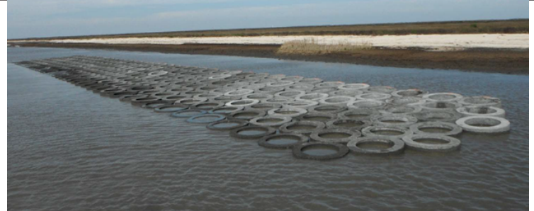
LA-08 project constructed along the Rockefeller Wildlife Refuge Gulf shoreline.
