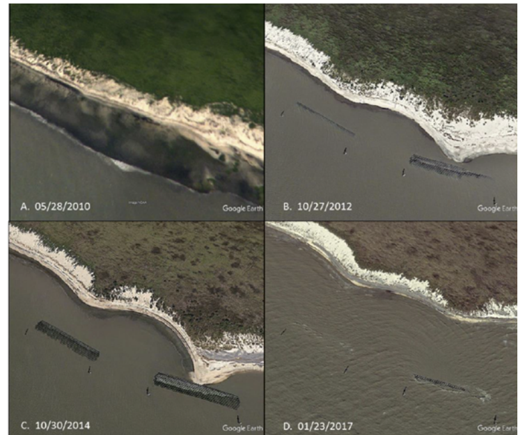
LA-08 project pre-construction (2010) and post-construction in 2012 (0.75 yrs), 2014 (2.5 yrs), and 2017 (5 yrs) Google Earth imagery.
