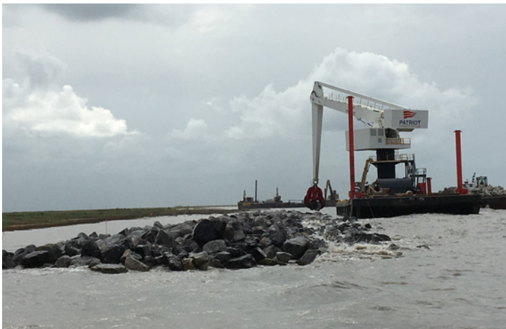
Constructing shoreline protection along the gulf shoreline of Rockefeller Wildlife Refuge.
