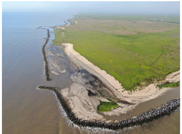
Shoreline protection breakwater constructed along the Rockefeller Wildlife Refuge gulf shoreline (LDWF aerial photo).
